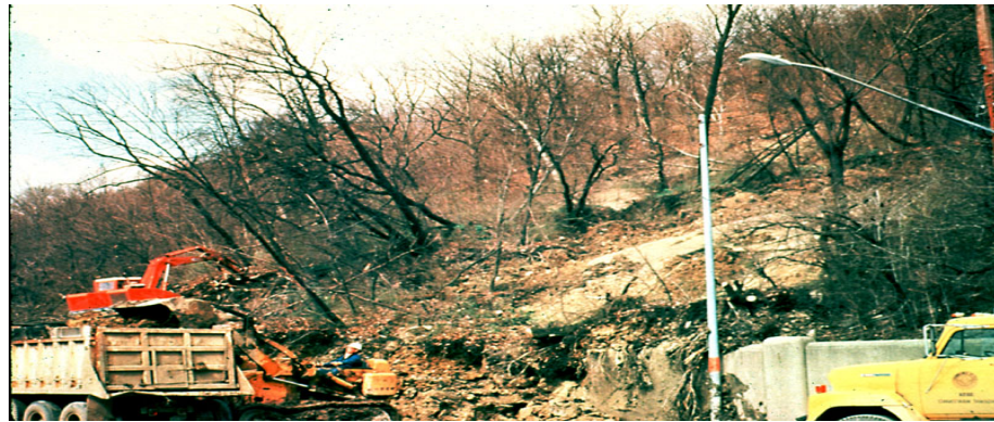
Cincinnati, Ohio ( http://landslides.usgs.gov/html_files/landslides/slides/slide8.htm )
