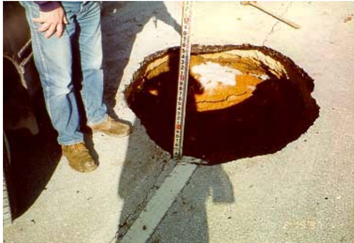
Sinkhole in Monroe County, WI ( http://www.uwex.edu/wgnhs/cavesink.htm )
