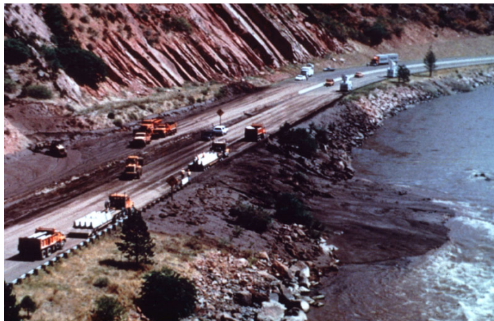
Landslide from fire damage in CO ( http://landslides.usgs.gov/html_files/landslides/slides/slide15.htm )
